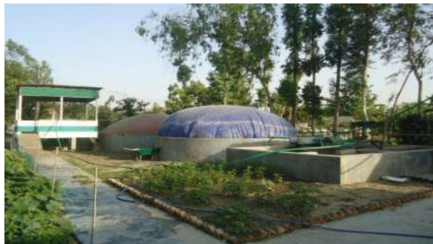
Community based Kitchen waste biogas plant in Gaibandha
